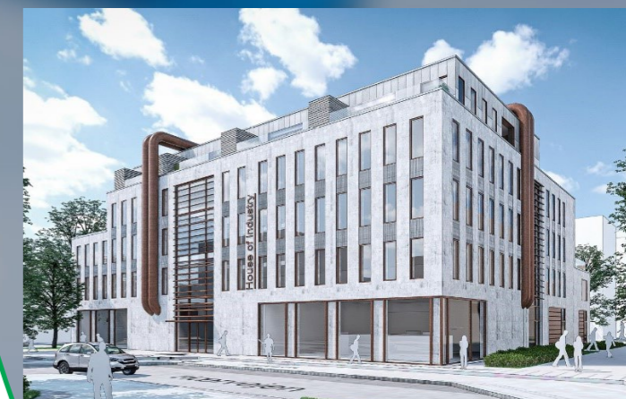
DEIF co-sponsors equipment at local mechanical engineering school.
